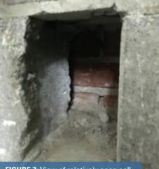
**FIGURE 7**: View of relatively open cell at CMU backup masonry and backside of face brick with open collar joint.
