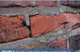
FIGURE 5: Cracks and voids at the mortar joints at the original brick masonry of the west facade
