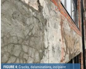
FIGURE 4: Cracks, delaminations, incipient spalls at exposed concrete frame and previous patching at concrete frame. Note the discoloration presumably due to moisture.
