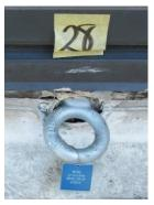
The objective of each test was to impose the the OSHA-required demands in each direction of use. All anchorages successfully passed the load testing and were marked with a WJE certification tag attached to the eyebolt.
